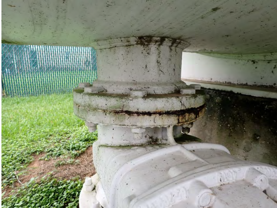
Photo 3: Inlet/outlet line with corrosion
