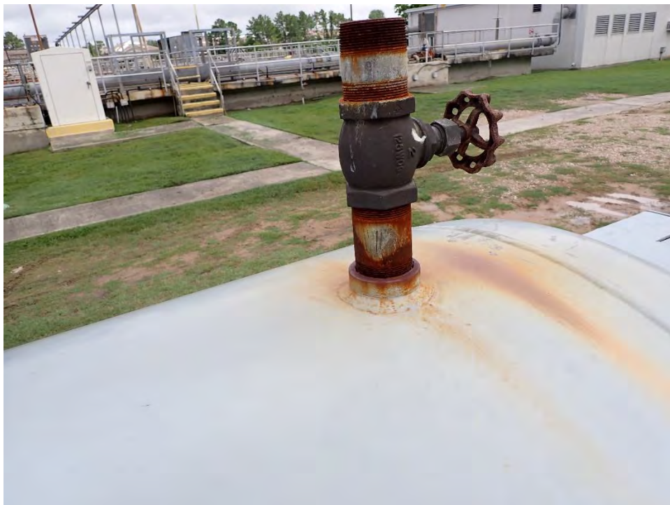
Photo 2: Air line with corrosion
