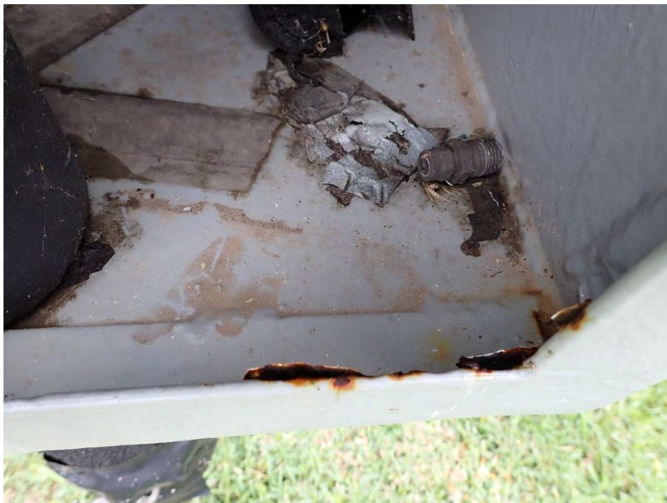
Photo 4: Equipment box with corrosion
