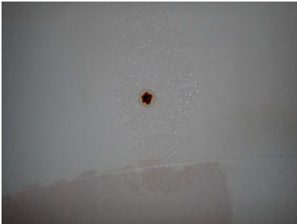
Photo 10: Interior penetration with corrosion
