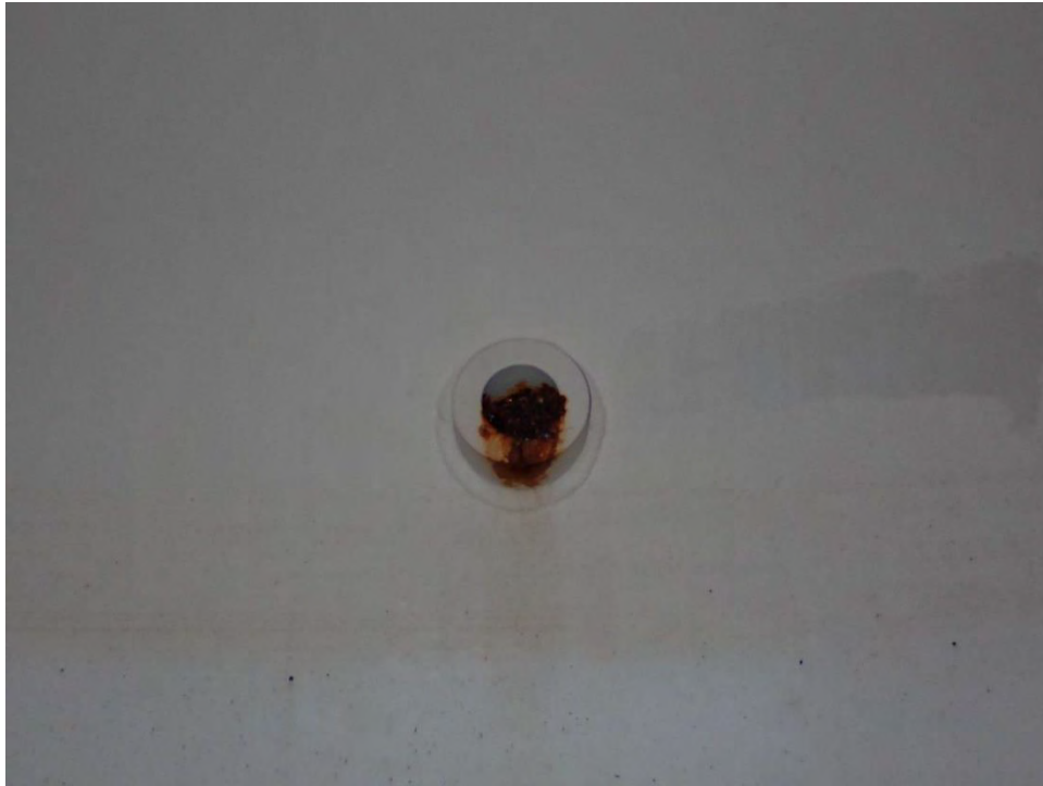
Photo 9: Interior penetration with corrosion
