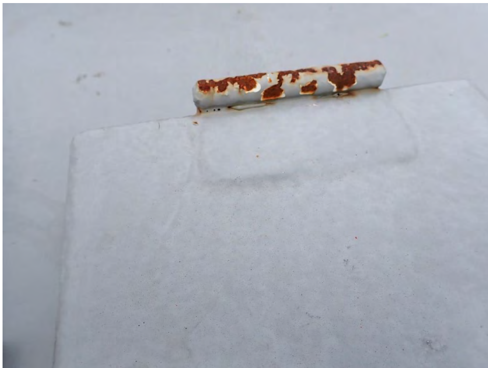
Photo 4: Equipment box hinge with corrosion
