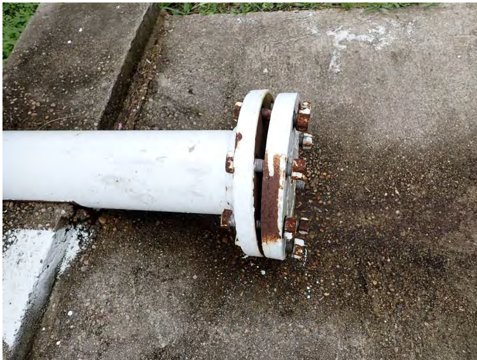
Photo 4: Drain line with corrosion
