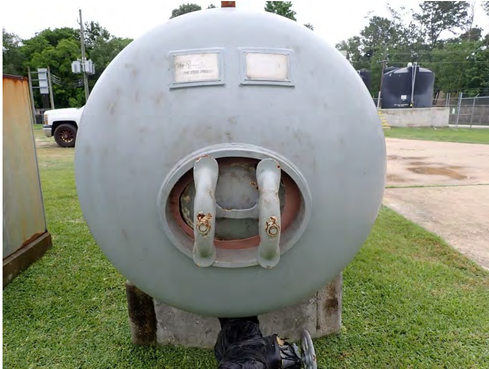
Photo 3: Elliptical hatch with corrosion
