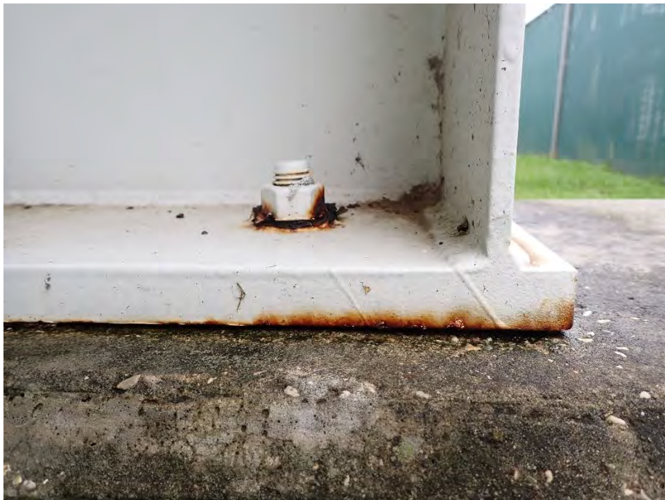
Photo 2: Tank saddle with corrosion
