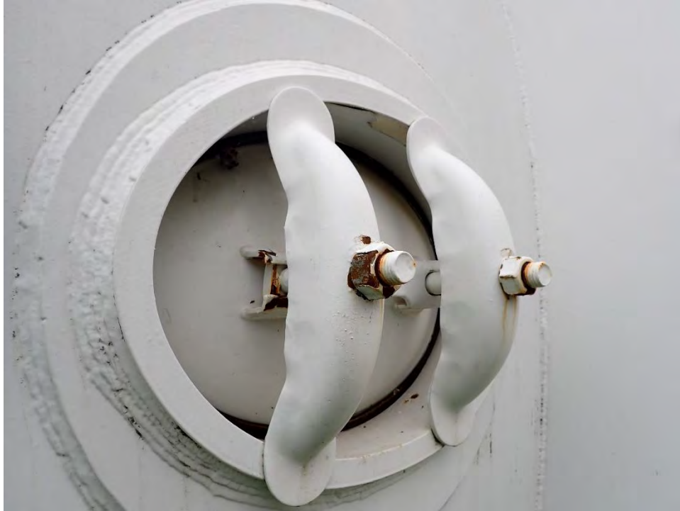
Photo 5: Elliptical hatch with corrosion
