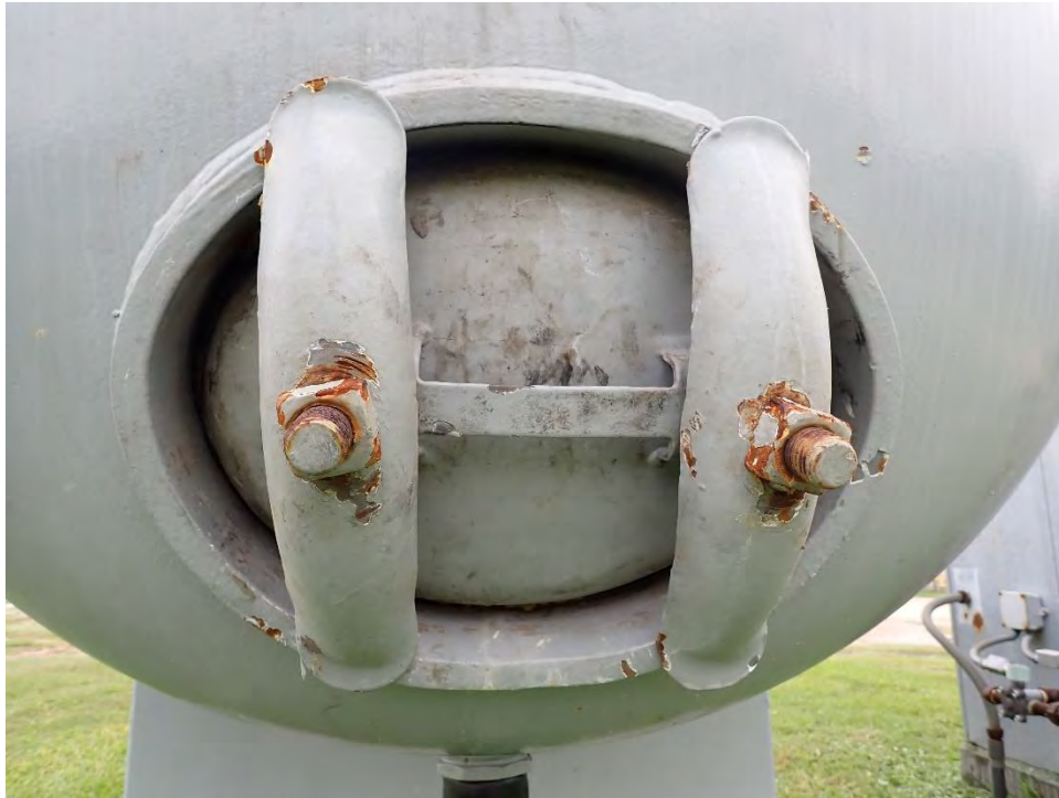
Photo 3: Elliptical hatch with corrosion
