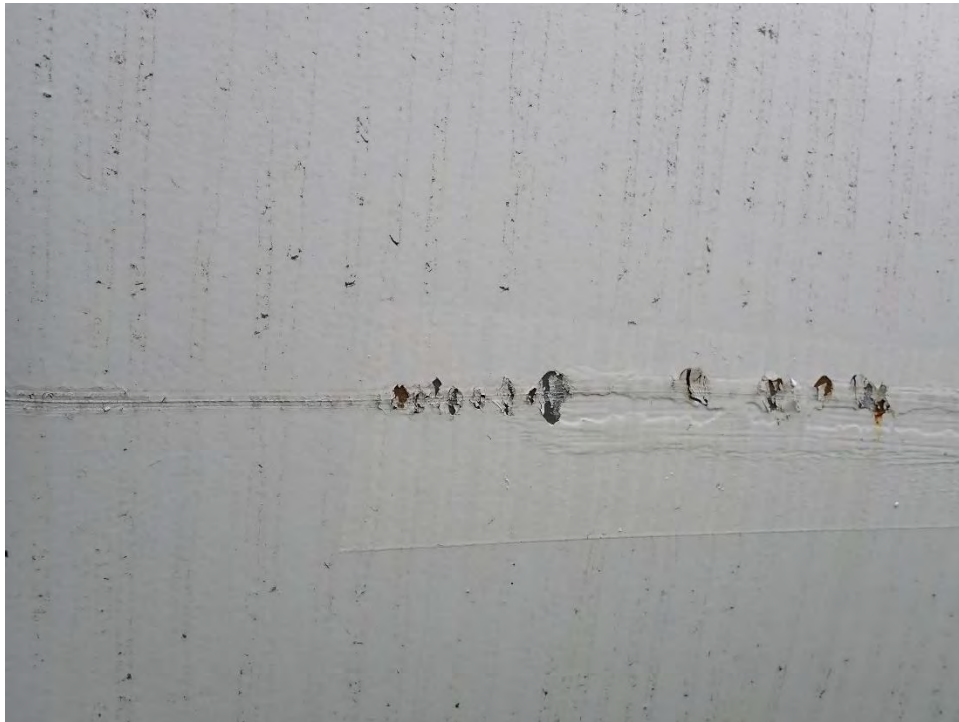
Photo 1: Tank shell with corrosion
