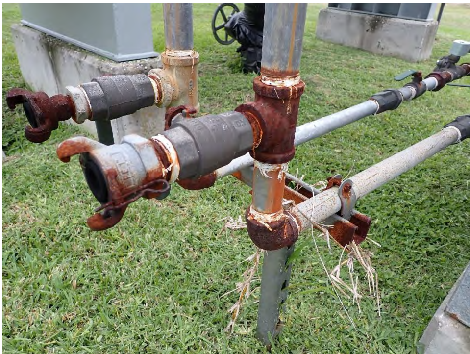
Photo 2: Crows foot with corrosion
