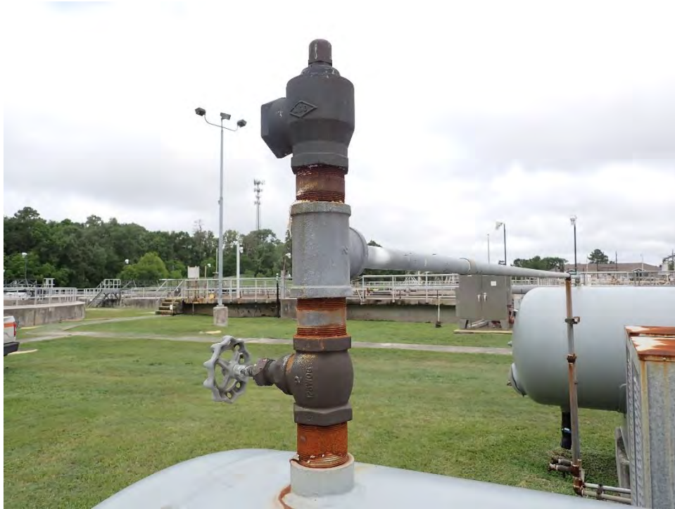
Photo 1: Air line with corrosion
